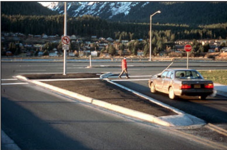
Crossing islands may be added to the middle of a street when the street is very wide.
