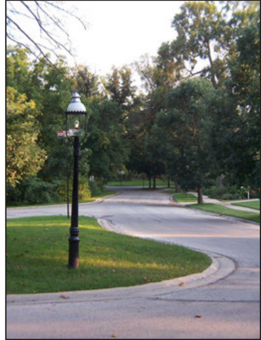
The serpentine street is a curving roadway that helps slow traffic through the use of curbs and landscaping.
