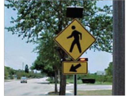
Activated, solar-powered, roadside RRFB at a mid-block crosswalk.
