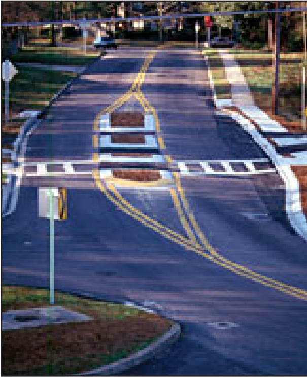
Crossing islands allow pedestrians to be concerned with one direction of traffic at a time. The roadway markings in the design shown here also help make motorists aware that a pedestrian may be crossing.
