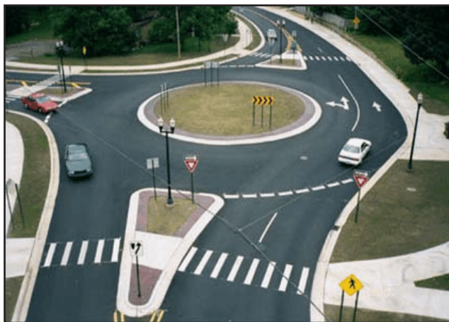
A traffic mini-circle helps reduce vehicle speeds, but still allows cars and emergency vehicles to pass through the intersection with little difficulty.
