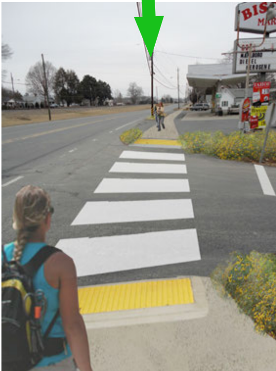
Creating a defined space for crossing both Hyde Street and the Biscoe Mart entrance for pedestrians along South Main Street would serve to capture the attention of motorists, making it safer for walking.
