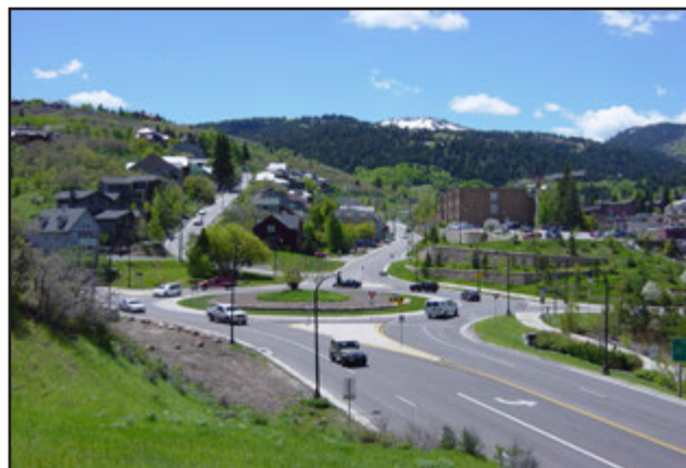
Roundabouts (and other circular intersection types) allow for landscaping, monuments, and other aesthetic uses within the central island.
