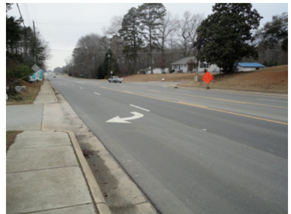
Lambert Road (top right in above picture) T's into West Main Street. With many destinations south of West Main Street, a pedestrian crossing treatment, with median island, high-visibility marked crosswalk, and signage would make this crossing more visible and safer.
