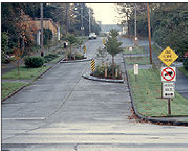
This chicane narrows the street to fewer lanes and requires traffic to move slowly.
