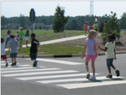
A variety of patterns are possible in designating a crosswalk; an example of a 'continental' design is shown above.
