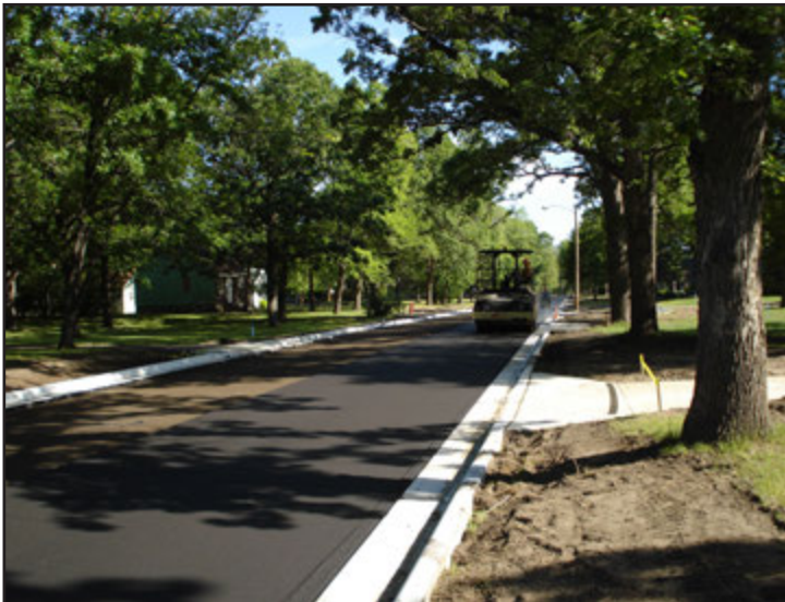
The landscaping on this street calms traffic by creating a visual narrowing of the roadway.
