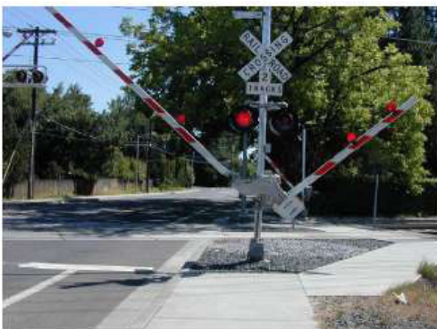
Examples of railroad pedestrian crossings with active warning devices.
