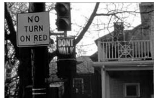
A low cost sign that restricts right-hand turns at a red light (Image from http://www.walkinginfo.org ).
