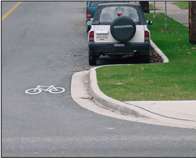
The curb extension makes motorists reduce speeds for turning and provides street parking.
