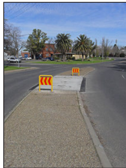
Crossing island allows pedestrians to stop before completely crossing a road.
