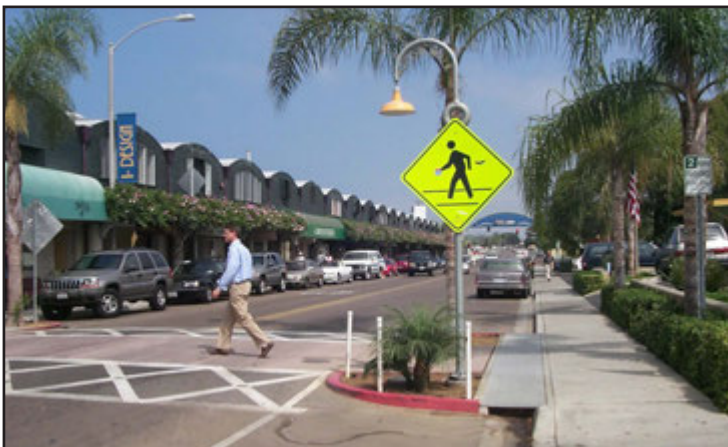
The curb extension narrows the width of the street and can be used in combination with crosswalk markings.
