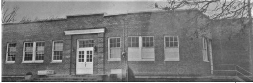
Former Peabody Academy built on the foundation of Douglas Hall. Douglas Hall's front stairs remain intact today. Photo Credit: Peabody Academy Facebook Group, photo date unknown
