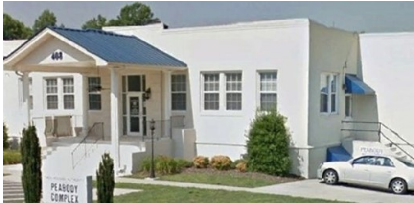
Former Peabody Academy, now used by the Troy Housing Authority
