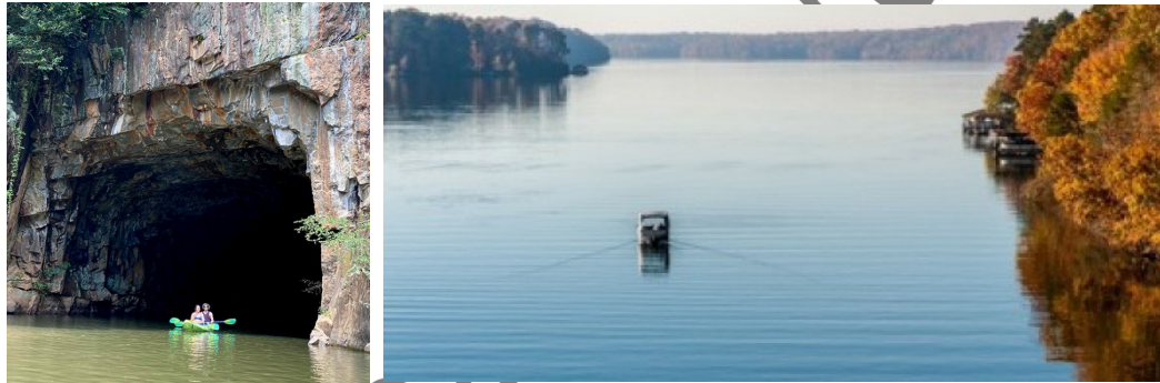
"Diversion Tunnel" at Falls Reservoir, Photo Credit: The Sway Insider's Guide to the Pines
